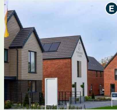
Construction of Florence Fields, a scheme of 226 homes developed by BCKLWN in partnership with Lovell, began in 2023.
