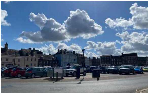
Figure 26. Existing parking at Tuesday Market Place compromises the setting of surrounding Grade II listed buildings
