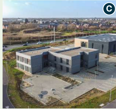
The King's Lynn Enterprise Park is a 15ha business park owned solely by BCKLWN, providing circa 48,000sqm of commercial floorspace with links to the A17, A47 a, A10 and mainline railway services to King's Cross.
