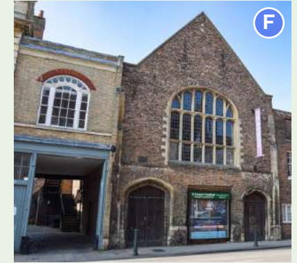
£30m renovation of St George's Guildhall & Creative hub has begun. It is the flagship scheme of the King's Lynn Town Deal Programme and priority of the Pride in Place Programme. The scheme has secured funding from the Shared Prosperity Fund, Historic England, and further public and private external funders.
