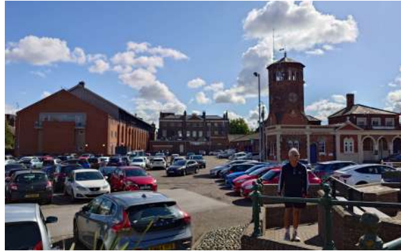
Figure 24. Existing parking at Common Staithe Quay compromises the setting of Grade II and II* listed buildings - Pilots Office, Baths building, Barclays Bank and Corn Exchange
